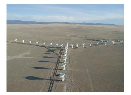
Figure 1.7: The 'Wye' of the Very Large Array(VLA) at New Mexico with 27 dishes making an effective dish of 4 km in diameter at its widest configuration *Image Credit: NRAO/AUI/NSF*
