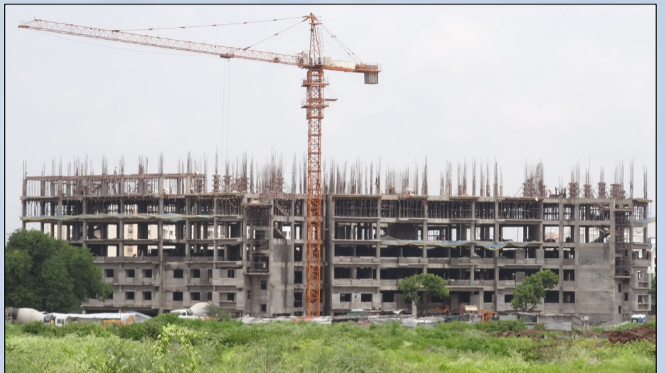
The 9-storey Student hostel, to be completed by 2012
