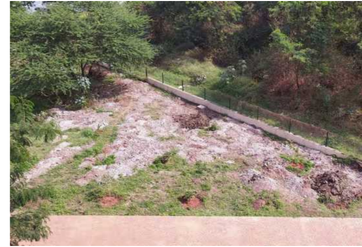
Construction rubble in front of Girls' hostel (Feb 15, 2020)
