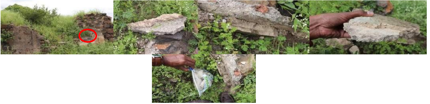
SAMPLE-2 (Mortar from Masonry of Merlons on Bastion)
