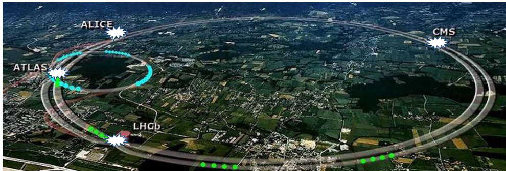
FIGURE 3.1: An aerial view the LHC ring with four collision points and corresponding experiment.
